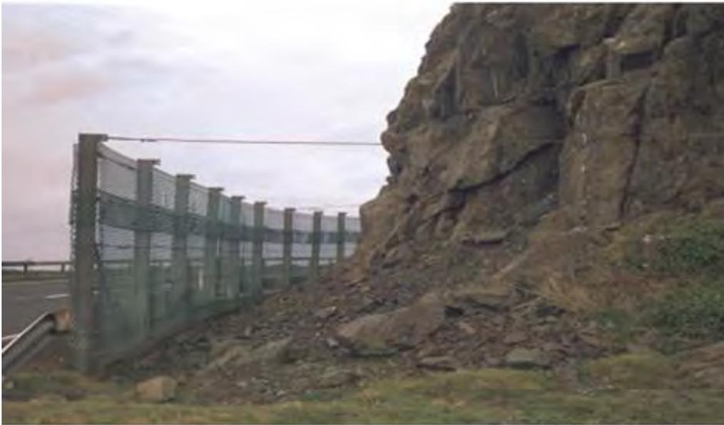
**Figure 6.10 Effective Rock Trap Barrier (A77, Ballantrae)**
